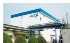
Fukuchiyama Plant: New Enzyme Production Building
